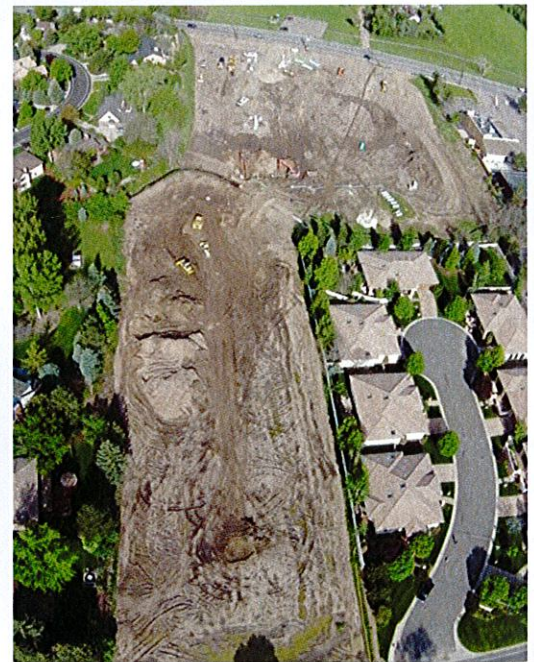
Wilder Lane under construction
