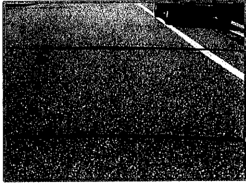
Transverse Cracks
