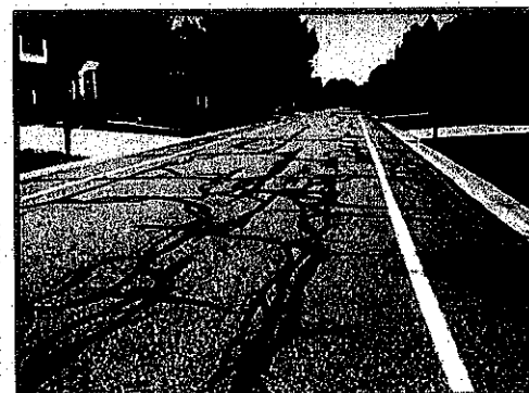
Shrinkage Cracks
