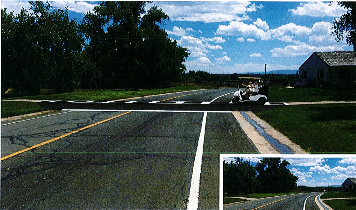
LOCATION 3 - CART PATH CROSSING ALONG FAIRWAY LANE
