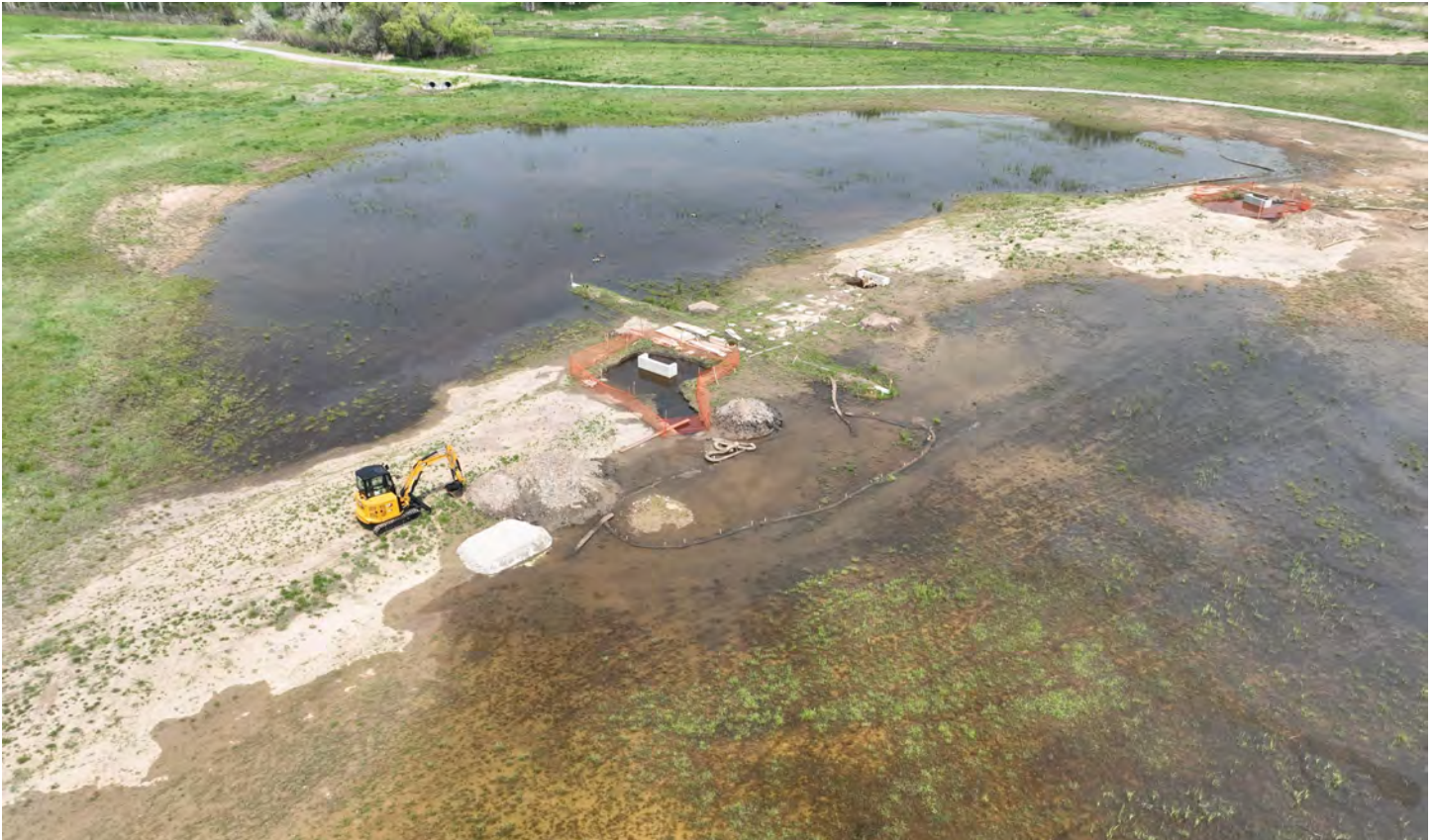
The boardwalk at the Wild Plum stormwater retention ponds after the recent heavy rains.
