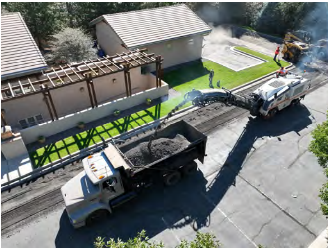
Paving the Town Hall parking lot.
