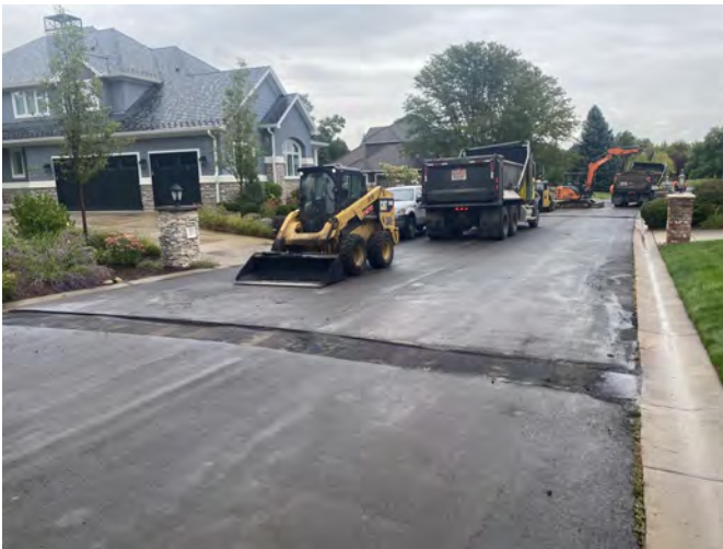
Repairing cracks on Arabian Place.
