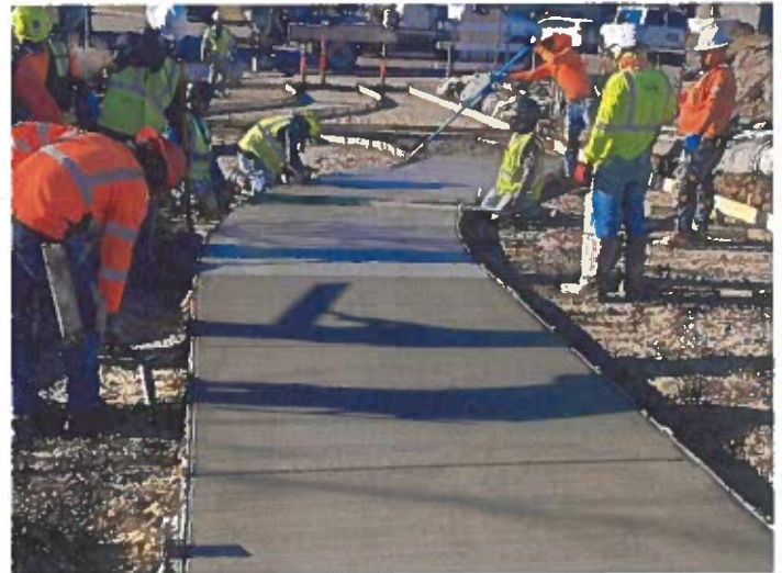
Top left: Digging trenches for the emergency access area in Wild Plum. Right: Paving the sidewalk for the emergency access area. Lower left: Metro Pavers repairing the last of the cracks in the Brookhaven neighborhood.
