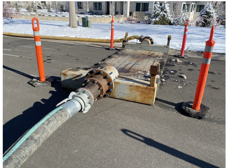
Sewer line repairs.
