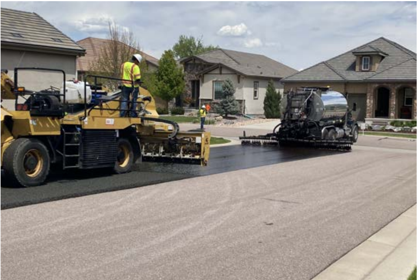
Applying chipseal to Aljor Street earlier this summer.
