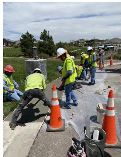
**Replace damaged gutter plans throughout Town.** The Town is in the final stage of a two-year initiative to replace ~100 gutter pans to improve drainage. Proper drainage helps protect drivers, pedestrians, roads, and foundations from water damage.
